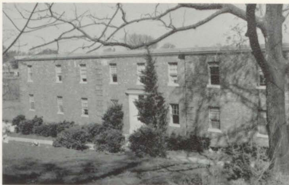
MILLER HALL: This fireproof dormitory was built in 1946 and accommodates about 75 cadets.
