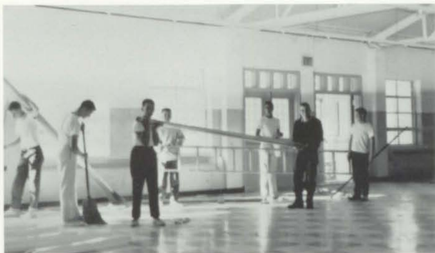
Moving in the new Mess Hall
