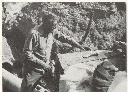
A HUGE CRATER IN THE "QUAD" WAS NOT THE START OF SWIMMING POOL CONSTRUCTION. TOM AND THE MAINTENANCE CREW WERE WORKING ON A STEAM LEAK.
